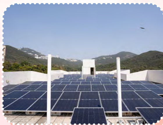
本會參與「賽馬會太陽能關懷計劃」，在康復中心大樓的天台安裝太陽能發電系統 The Society participated in the 'Jockey Club Solar Care Programme' and installed a solar power generation system on the rooftop of our rehabilitation centre
