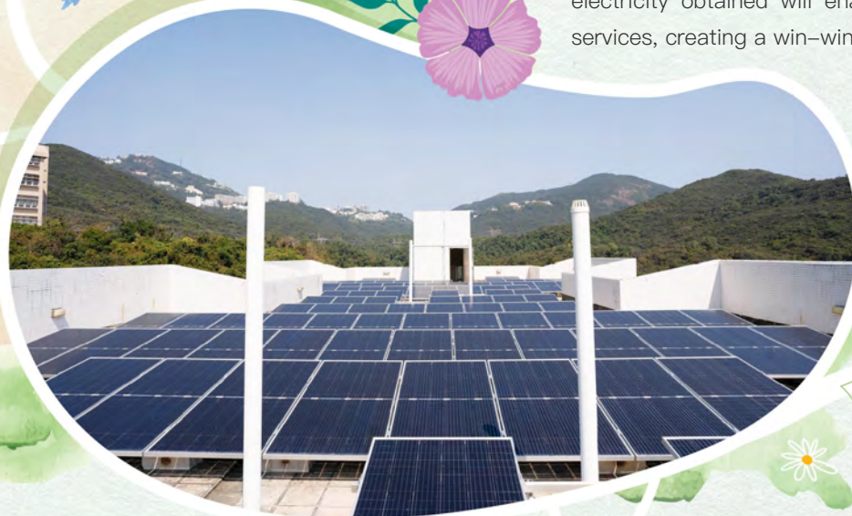
每塊太陽能板均朝向南方以務求攝取最高的太陽照射力 Each solar panel faces south in order to obtain the greatest amount of solar power
